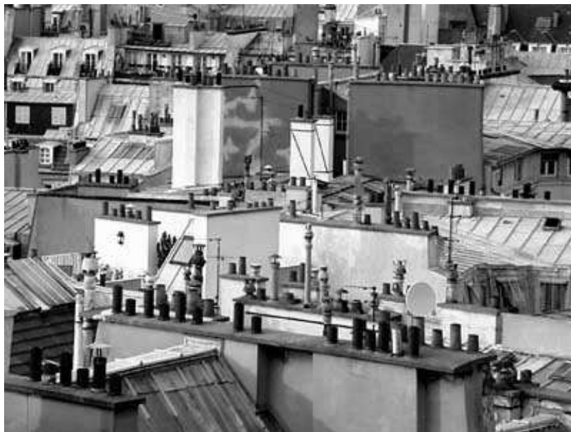
Figure 4.54: Roofs of buildings in an urban area.
