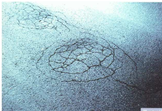
FIGURE 2.6. Faiençage circulaire [LCPC, 1998]
