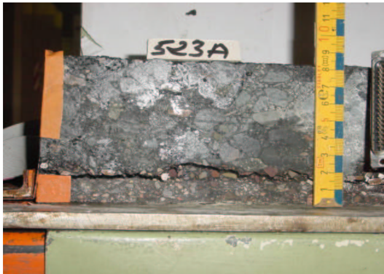
FIGURE 5.31. Propagation horizontale partielle de la fissure
