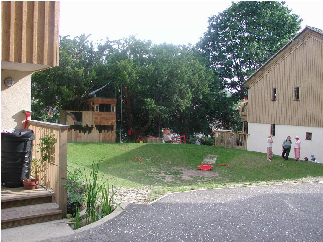
Photo 3: Photo the Stroud “Alternative” housing project. An swallow infiltration basin is used as a play ground (a Bob Bray project).
