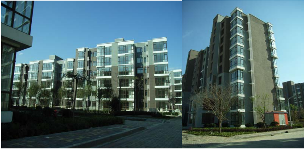
Figure 8-1 Completed medium-rise residential buildings in HXJD project
