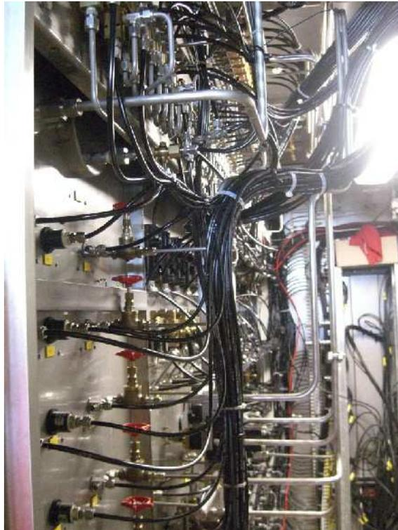
*Illustration 19: The inside of a control panel. Each set of cables or pipes corresponds to an indicator on the front of the panel. Photo: courtesy of GDF Suez Production Nederland B.V.*
