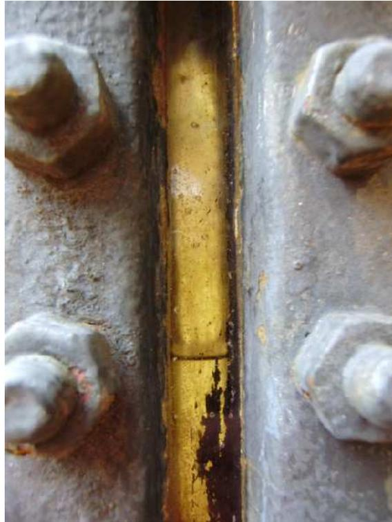
*Illustration 12: A sight glass. The horizontal line indicates the interface, in this case, of condensate (top) and water (bottom). Photo: courtesy of GDF Suez Production Nederland B.V.*
