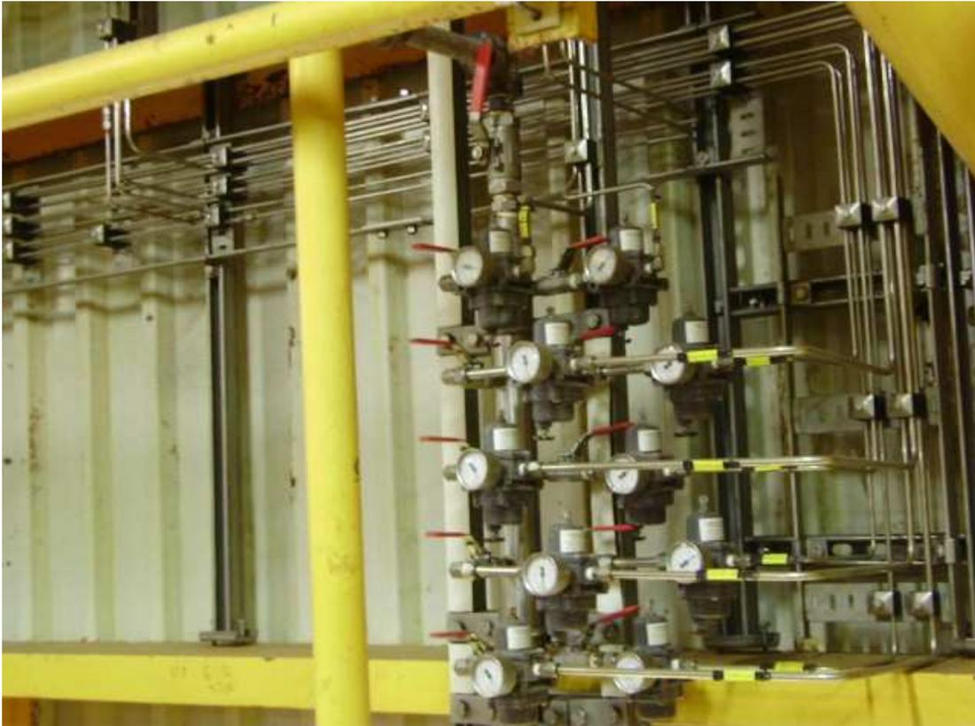
*Illustration 16: Tubing in the way, partially blocking view of gauges. Photo: courtesy of GDF Suez Production Nederland B.V.*
