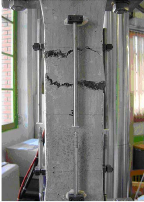
Figure 1.21. Multi fissuration du CEMTEC® en traction directe.
