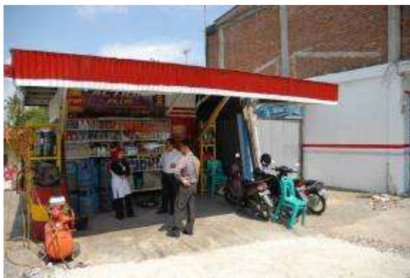
Construction of a gas station
