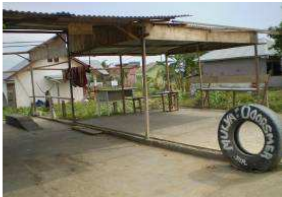
Construction of a car washing area
