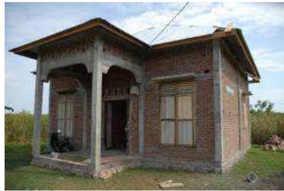
Progressive construction of a house
