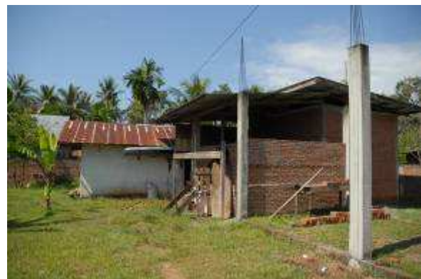
Progressive construction of a house
