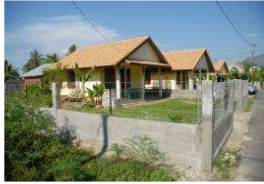
Construction of a fence
