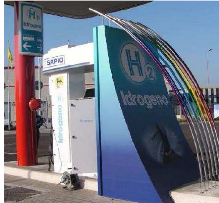
Figure 4.12 Zero Regio hydrogen refuelling unit in Mantova Source:
