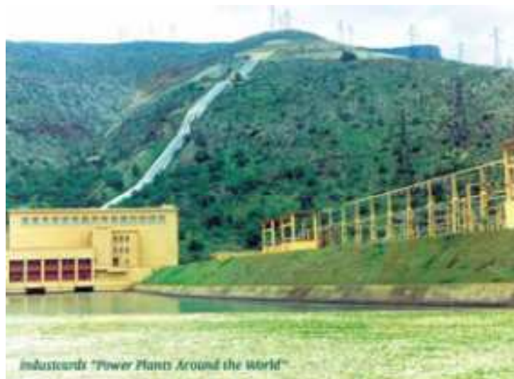
Figure 7.3 Lower water reservoir
