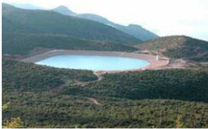
Figure 7.4 Higher water reservoir
