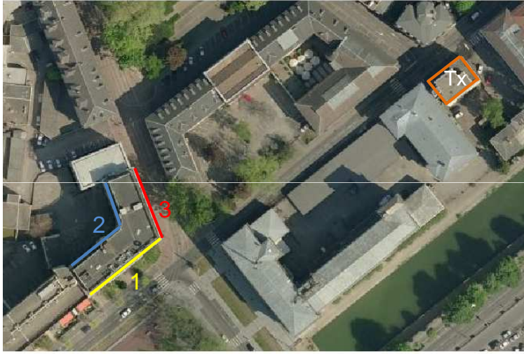
Figure 4.8: Aerial photos showing reception building facades with different propagation conditions.
