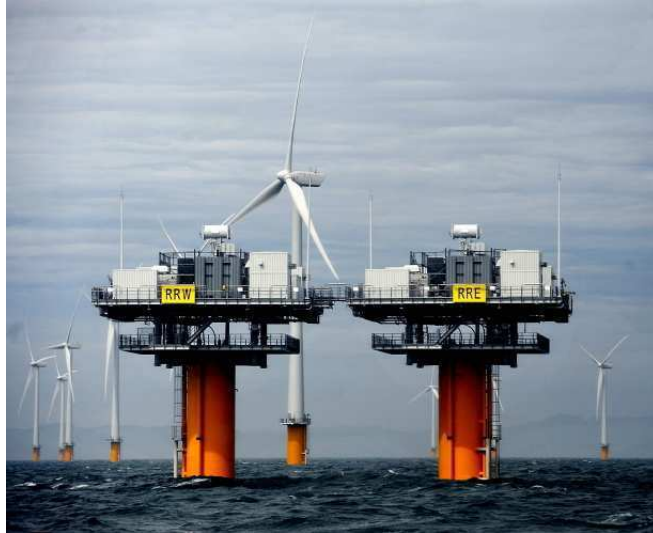
FIGURE 1.31 – Station offshore de la ferme offshore Robin Rigg, 180 MW (Crédit photo E.ON)
