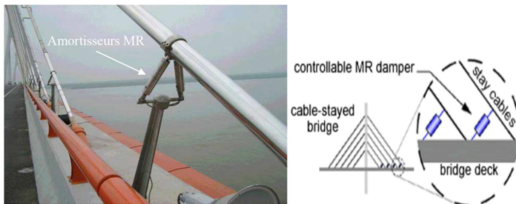
Figure 1.6 – MRF in Dongting bridge in China (after J.M., Ko, Y. Q., and Ni, [13]).
