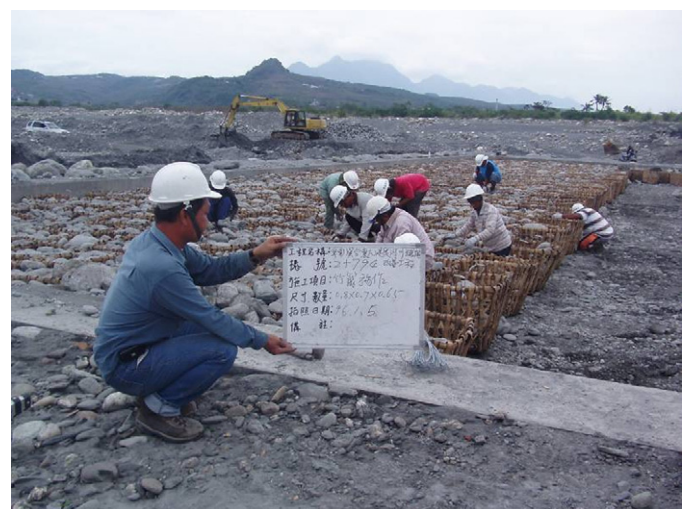
Fig. 2. Bamboo gabions currently used in Taiwan. (Photograph courtesy of Rui-Lin Chen, WRA Taiwan).
