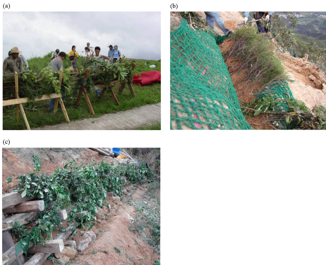
Fig. 4. (a) Live fascines were constructed on-site using Ficus microcarpa and Salix babylomica species. (b) Brushlayers were installed using Gardenia jasminoides and Melastoma candidum species and (c) live cribwall was installed using Gardenia jasminoides and Melastoma sanguineum , Phyllanthus emblica , and Rhodomyrtus tomentosa species at Cloudy Hill, Hong Kong, China. (Photographs courtesy of Manusell AECOM, Hong Kong.)
