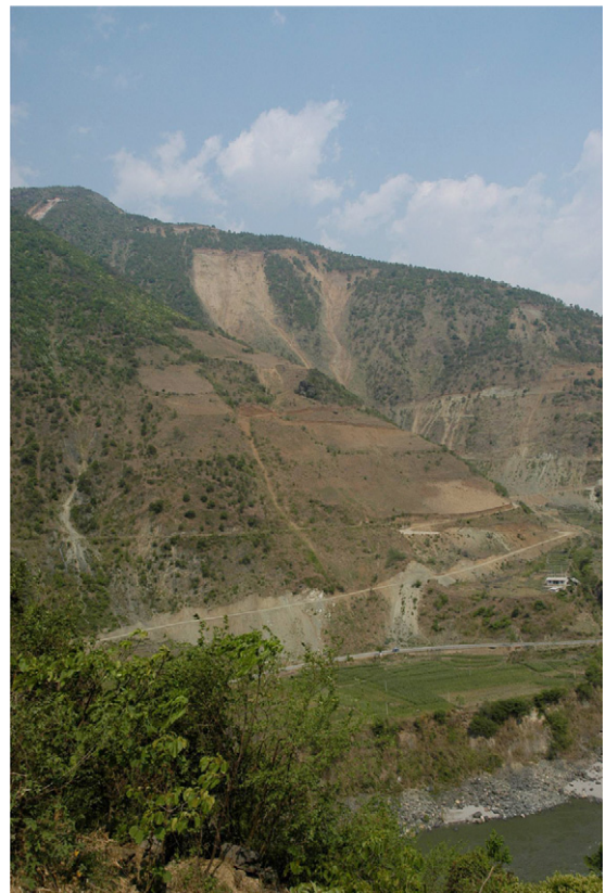
Fig. 5. Recent accelerated construction of roads linking villages and towns have resulted in all the landslides and erosion visible at this site in the Yunnan province, China. Soil is entrained downslope, resulting in sedimentation of the river Salween (bottom of image), a UNESCO World Heritage Site.
