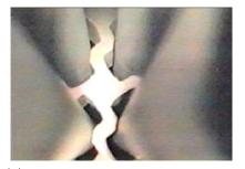
(b) Clean SG tube and support plate with flow paths.
