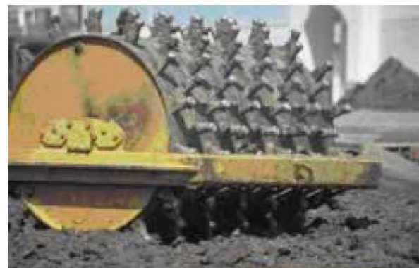
(f) Compaction with vibratory padfoot rollers
