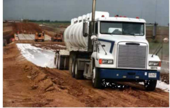
(b) Spreading lime
