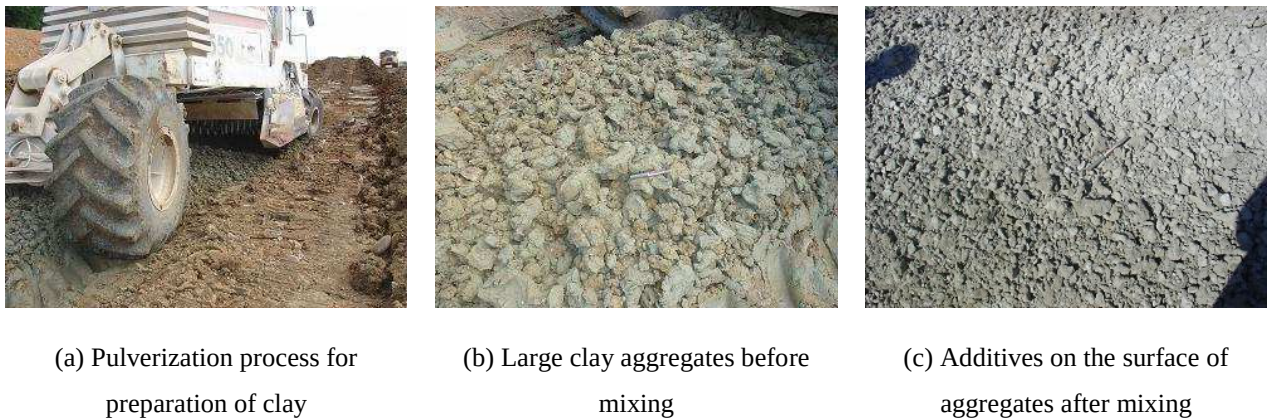
Figure 5-46 Field preparation and storage at a site near the experimental embankment
