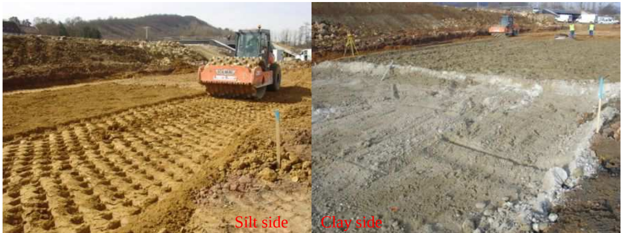
(a) Silt side in construction
