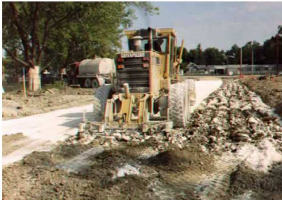
(c) Scarification after spreading
