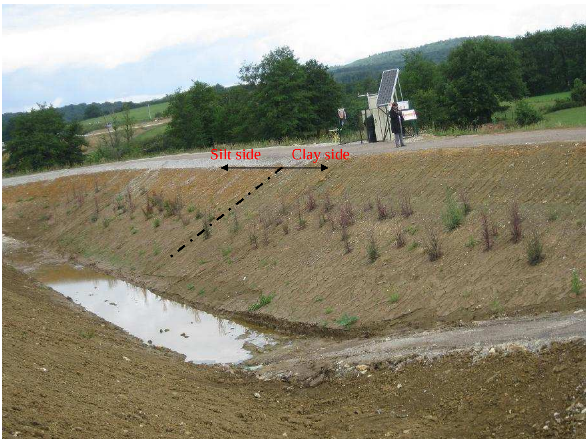
(c) Experimental embankment after construction
