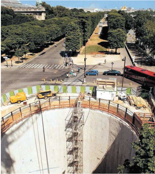
Figure 1. 88: Centrale (photo Solétanche Bachy).
