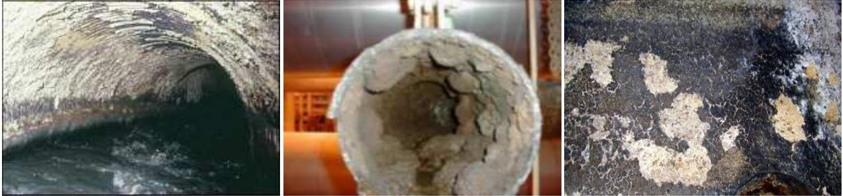
Figure 1.2: Examples of MICC of sewer pipe
