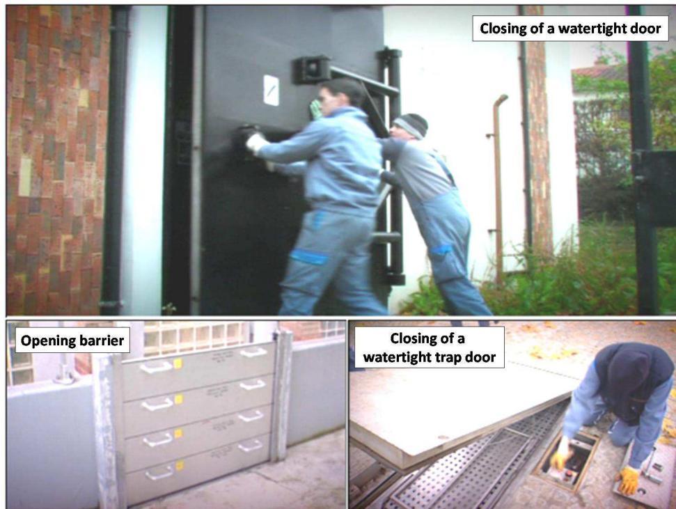
Figure II.1-6: Example of techniques used in Val-de-Marne to protect installations (Source: Snapshots from the video: 'Ohval! 18 Spécial crue centennale' http://www.cg94.fr/webtv/term/1061#19442 )
