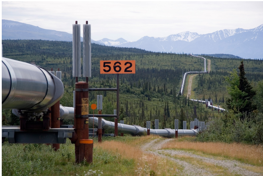
Figure I.15 – Pipeline Trans-Alaska muni de caloducs ailettés [7]
