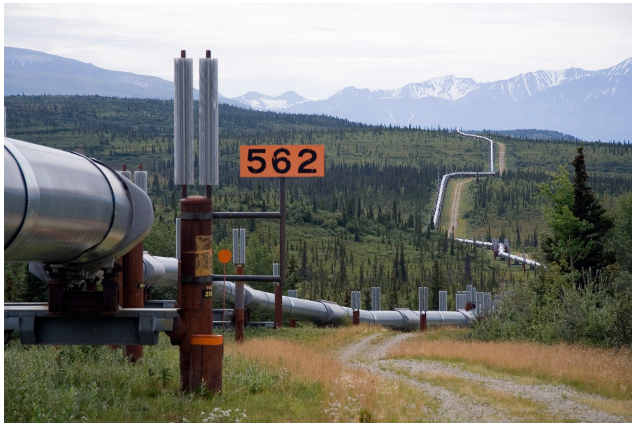
Figure I.15 – Pipeline Trans-Alaska muni de caloducs ailettés [7]
