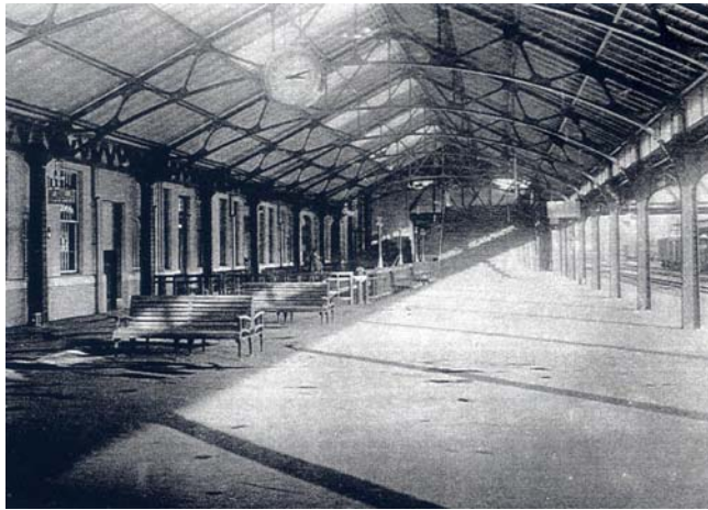
Figure 858 Abri de quai
