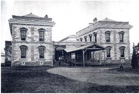
Figure 670 Gare de Shinbashi (1871)
