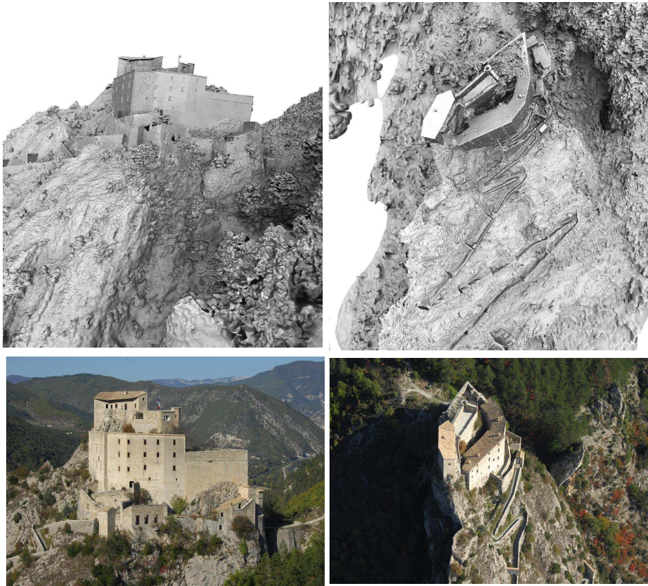
Figure 4.12: Results on Entrevaux data set. Top row: final model of Entrevaux. Two bottom rows: 2 images in similar views (© IMAGINE/CSTB).
