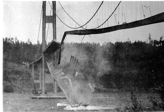
(b) failure of the bridge
