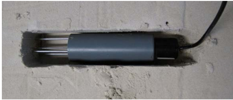
Fig. 3.2. Installation of ThetaProbe
