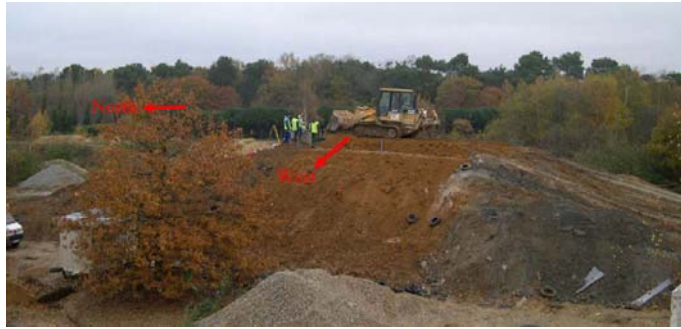
Fig. 1.48. The photograph of the experimental embankment in Rouen (Cui et al., 2010)
