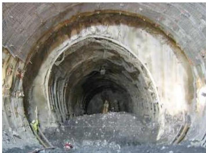
**Fig.4.** Large anisotropic convergence at chainage 1,340 (after Mathieu 2008)
