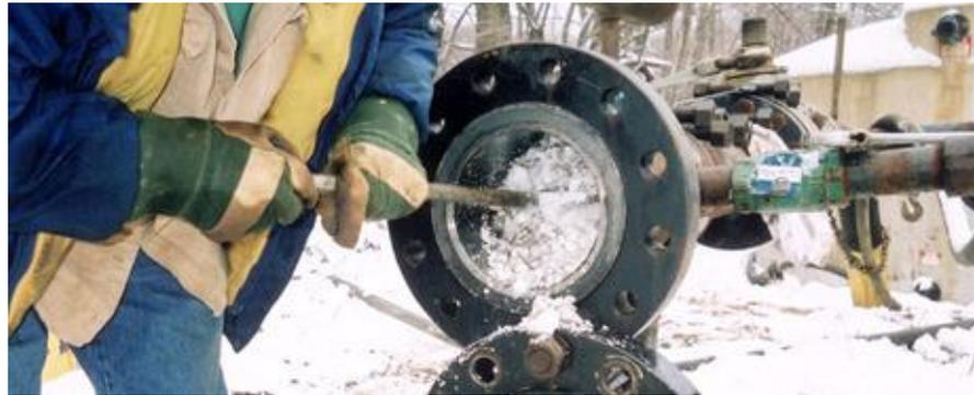
Figure 1.17: Gas hydrates removed from a pipeline [1.41]
