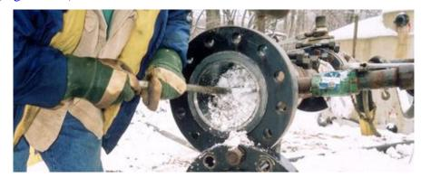
Figure 1.17: Gas hydrates removed from a pipeline [1.41]
