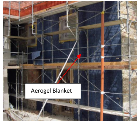
Fig. 1.10: Aspen aerogel insulation for retrofitting of an old brick dwelling
