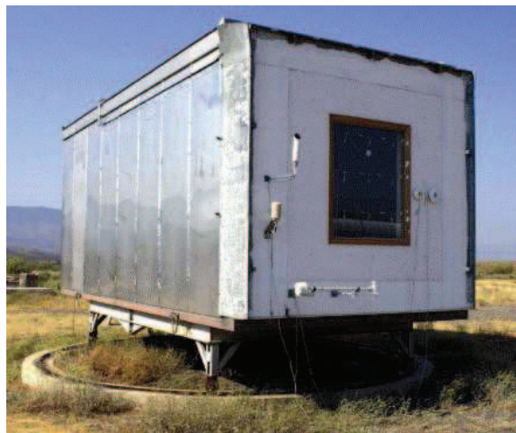
Figure 12 : Cellule test PASSYS [31].
