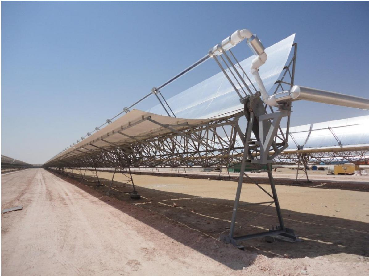
Fig. 1.1: Picture of the parabolic troughs of Shams 1, a CSTE power plant located in the UAE. © Yehia Eissa, 2012.
