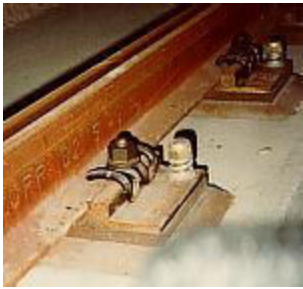
(a) Fastening system with resilient pads from Tiflex of UK (rail pad and baseplate pad)
