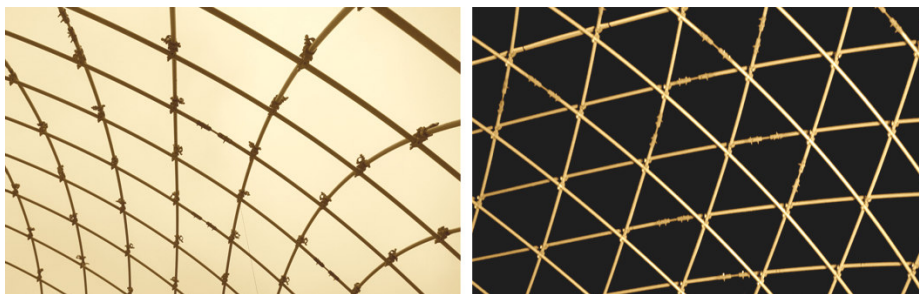
Figure 1.5 - Triangulation du gridshell
