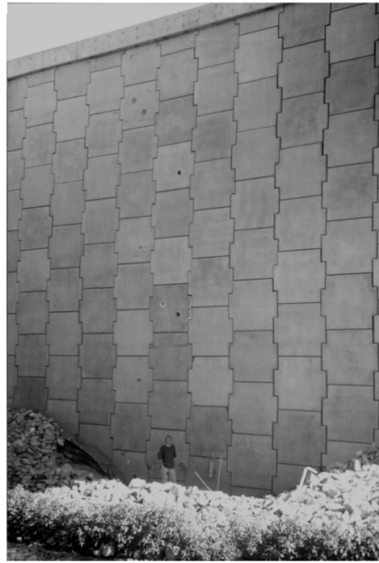
Figure 1-13 : Mur de Minnow Creek, Indiana, USA [RUN01]
