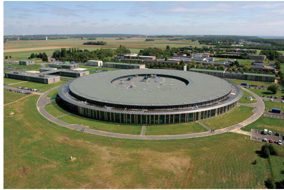
Figure 2.20: Picture of the SOLEIL synchrotron [65].
