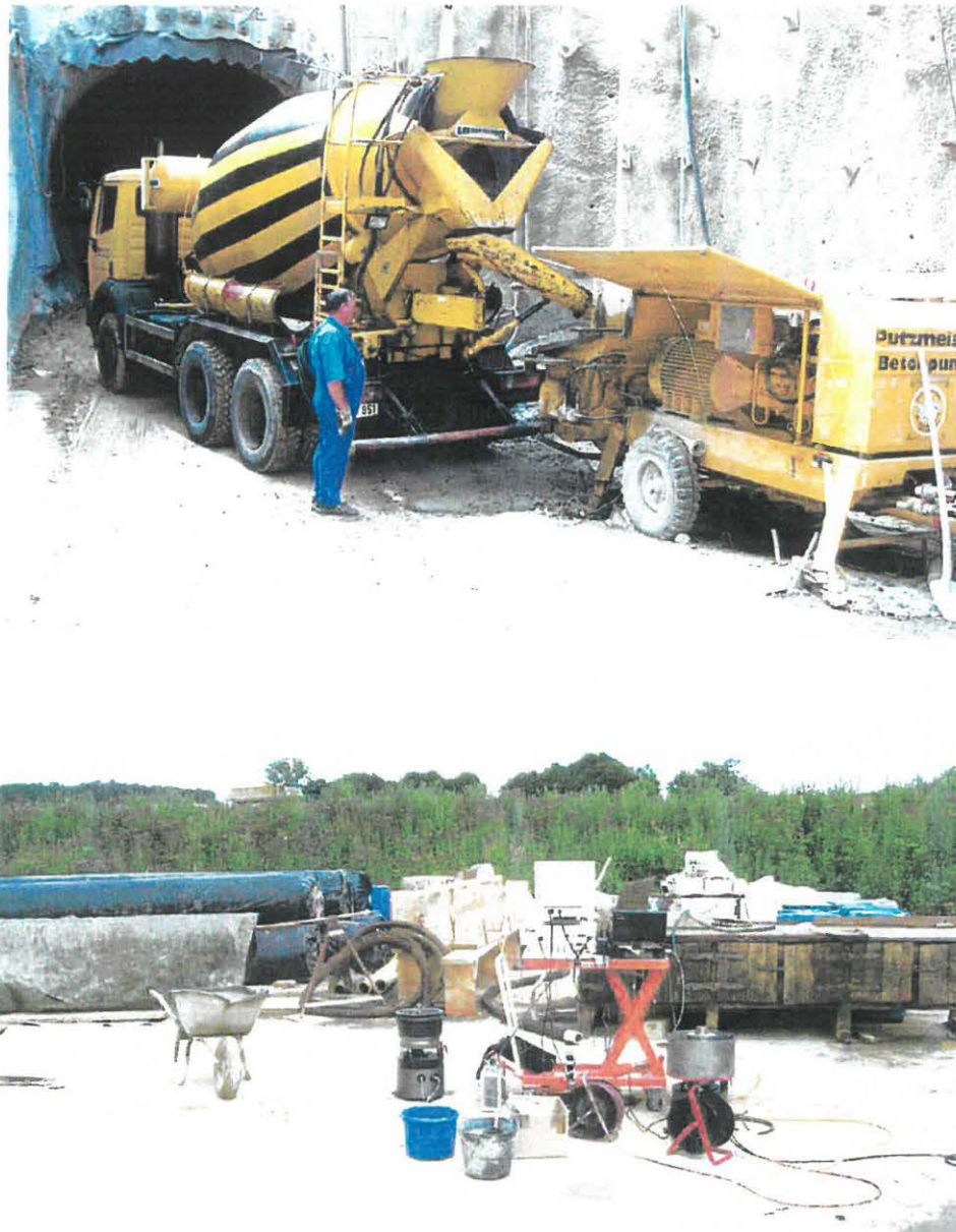
Figure VII.5 – Chantier de Pforzheim.
