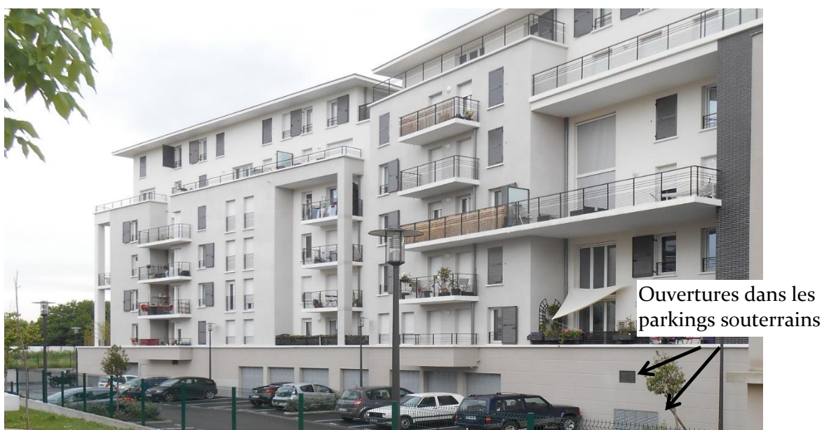
Figure 56 Parc-en-Seine, Villeneuve-le-Roi Source: Adeline Duport, 05/2014
