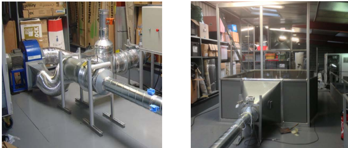
Figure 1. Experiment layout: ventilation system (left) and test chamber (right)
