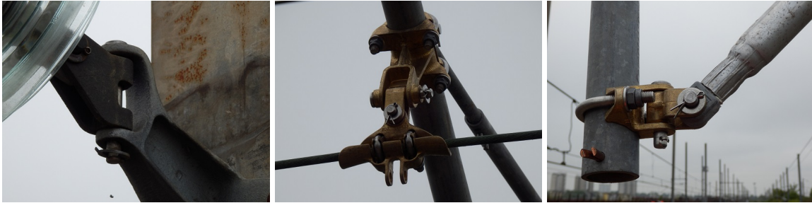
Figure 1.5: Mechanical bounds between bracket and mast (left), MW and mast (center) and registration arm and SA (right)
