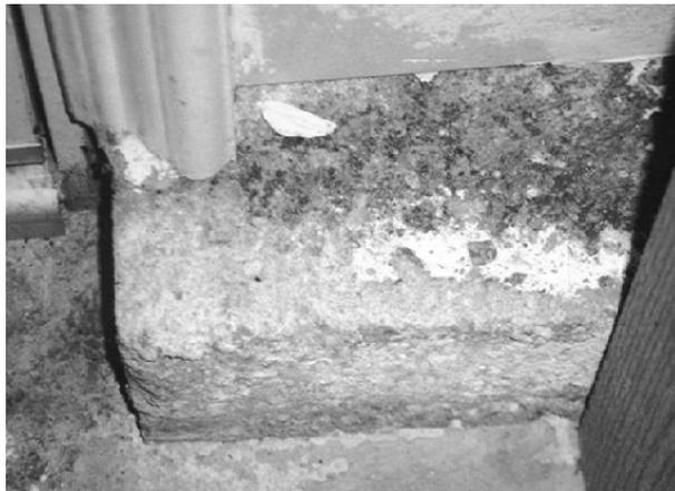
Figure 1.1: Foundation of residential house in California, attacked by sulfate-rich ground waters. The attack caused volumetric expansion, spalling, and efflorescence. Pictures credit: J. Skalny.
