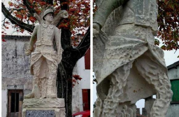
Figure 1.7: An example of salt-induced damage which has been recognized in the statue of a soldier in La Rochelle, France. Photo credit: Rob van Hees.
