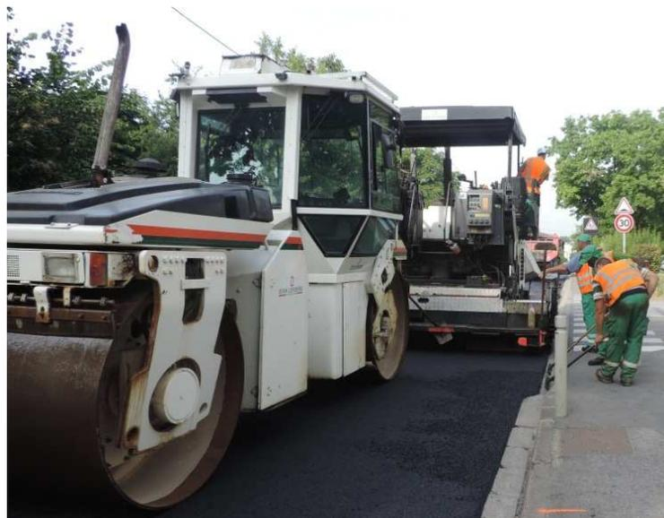
Figure 9 : Compactage (Chantier Eurovia)
