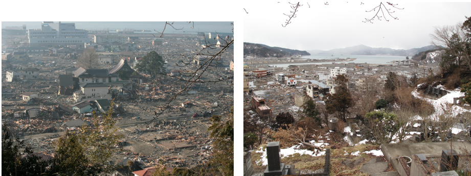
Figure 1: Introduction - Pictures from the NOAA website ( http://www.ngdc.noaa.gov/hazardimages/event/show/256 ) of the Otsushi city in the wake of the March 2011 tsunami.
