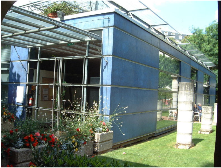
Figure 3.2: Picture of the LUSAGE living lab's building in Paris (France)
