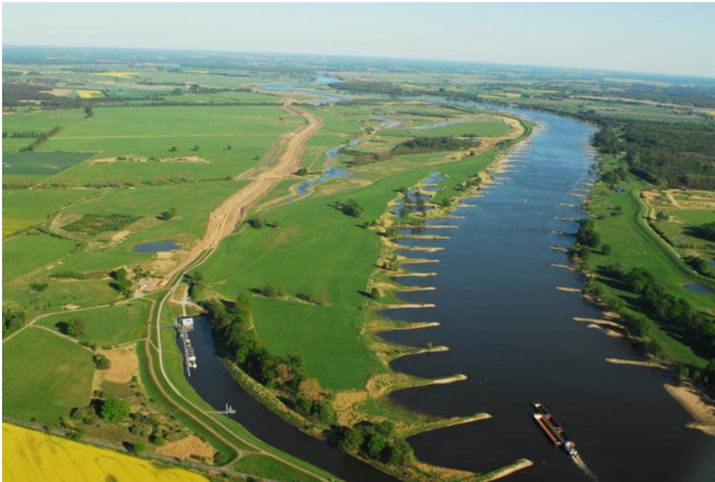
Figure 8.2: Photo of Elbe river, looking upstream from the harbour of Lenzen. Construction phase of the dike relocation. Photograph taken by J.Purps, 2007-04-29
