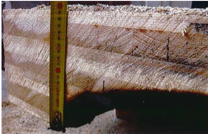
Figure 6.1: Reduced cross section of Test-1 after the fire exposure
