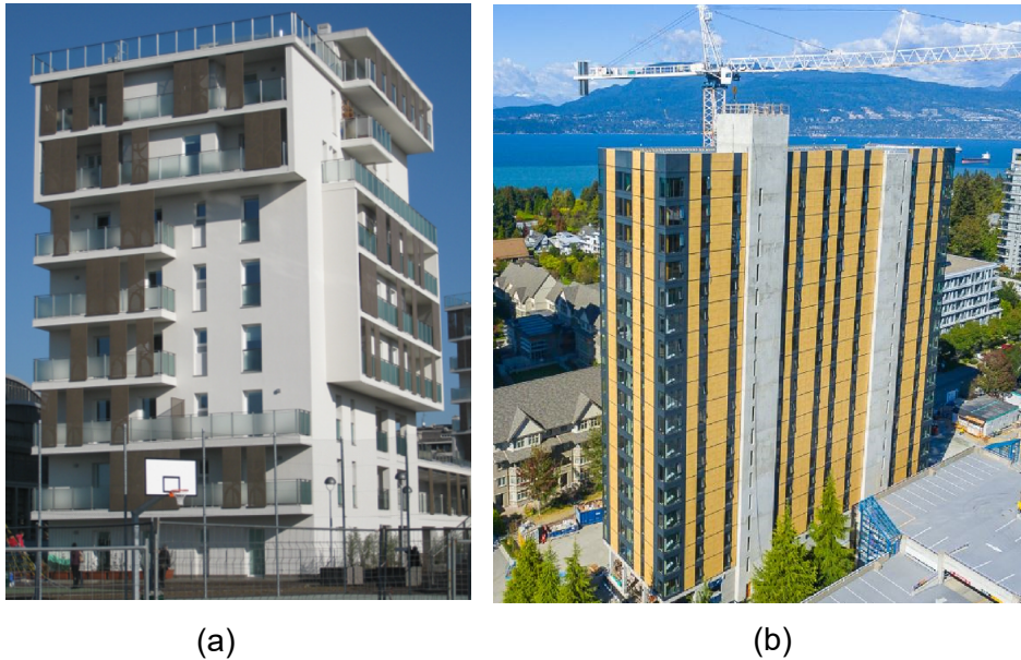
Figure 1.2: Tall CLT buildings: (a) 9-story building in Milan (Bernasconi 2016) and (b) on-going project in Vancouver of a 18-story building with concrete cores (Fast et al 2014)
