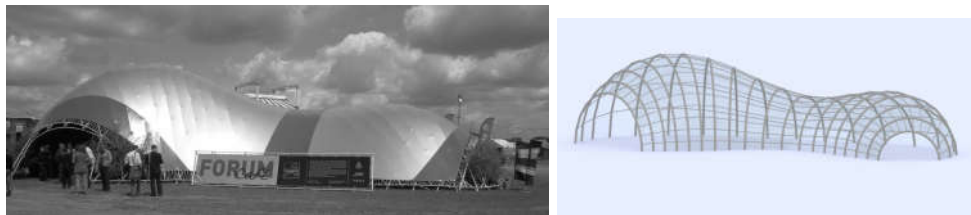
Figure 4.37 – The ‘peanut’ gridshell of the Solidays forum: built project and interpretation with the inversion of a surface of revolution.
