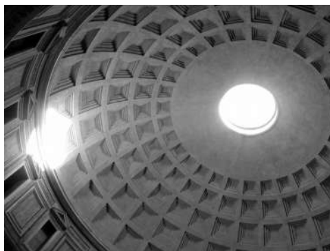
Figure 2.2 – The pantheon in Rome, a concrete shell as a surface of revolution ( picture: Romain Mesnil )
