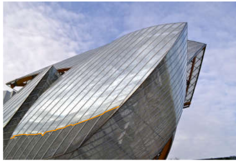
Figure 2.12 – The Louis Vuitton Fondation: the panels have a cylindrical shape, yielding non-smooth reflections light orange curve highlighted by us (picture: Romain Mesnil)
