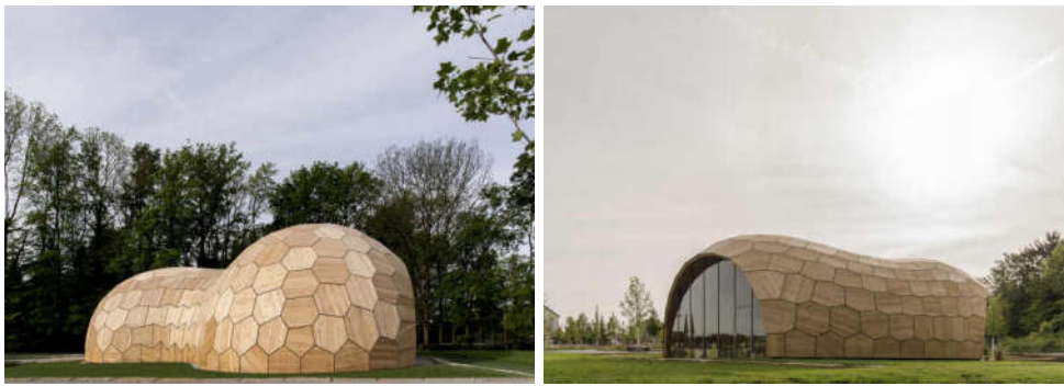
Figure 2.14 – Fortspavilion: a plated shell structure covered with planar hexagons ( picture: ITKE Stuttgart ).
