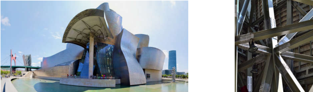
Figure 1.3 – A complex shape can hide an inefficient structure (picture: Romain MESNIL)
