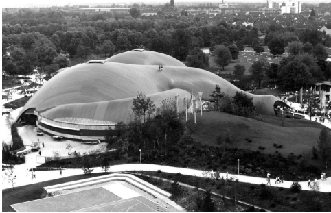
(a) Mannheim Multihalle (archive Frei Otto)
