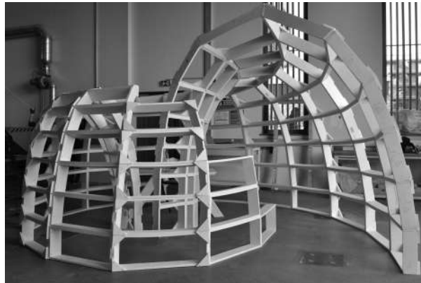
Figure 4.42 – A pavilion built with torsion free-nodes on a super-canal surface.
