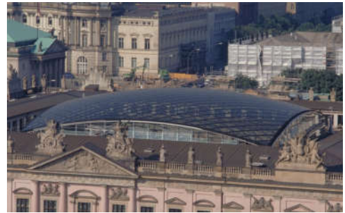
(b) Gridshell covering the court of the Deutsches Historisches Museum picture: SBP
