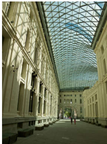
Figure 1.5 – The gridshell covering the courtyard of the Palacio de Comunicaciones ( picture distributed under Creative Commons licence )
