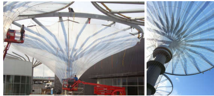
(a) Membrane structure during installation (picture: LEICHT GmbH) (b) Membrane structure after completion (picture: Romain Mesnil)
