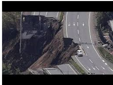
Figure 6.31 – Landslide triggered by the earthquake.
