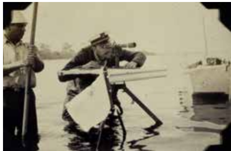
Figure 2.1 – Operator manipulating a plane table. Courtesy NOAA.
