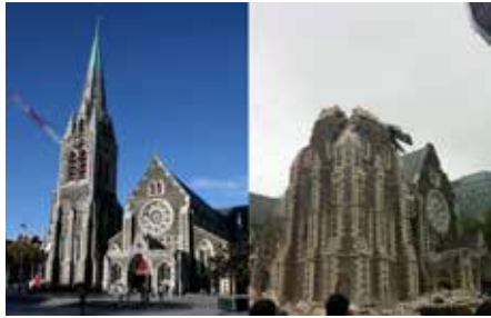
Figure 6.28 – Collapsed bell tower.
