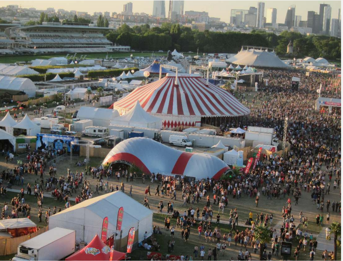
1.17 Solidays GFRP gridshell built in 2011 in Paris, France
