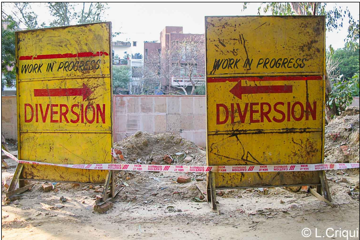
Photo 1/D. Work in progress (Delhi, 09/02/2013)
